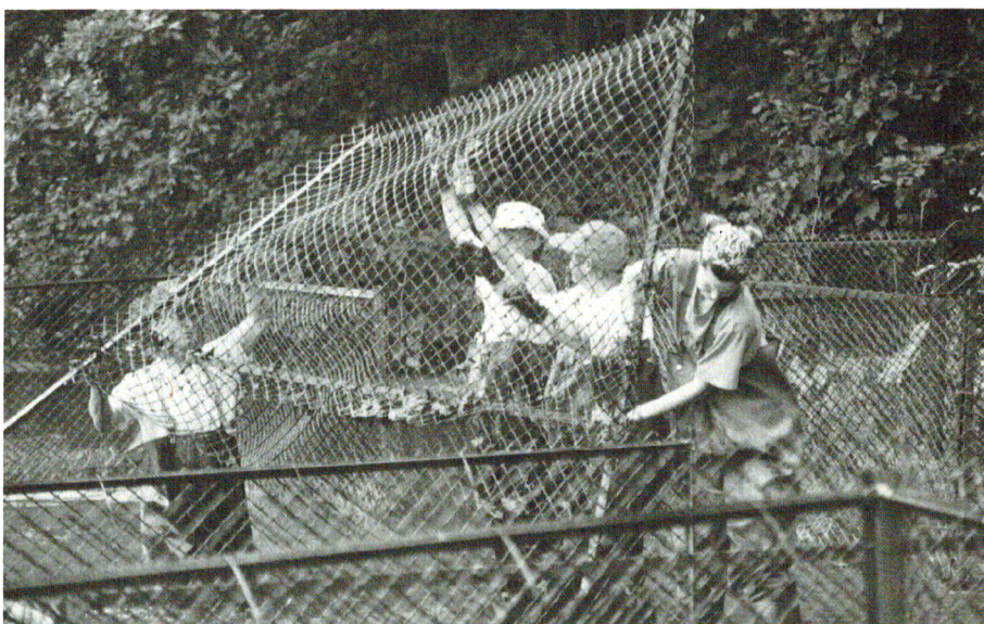
Eight-foot by eight-foot exclosures are built of four panels of weld-wire or plastic snowfence mounted with cable ties on T-bar frames. Volunteers construct the single panels on a board walk, and then carry them out into the marsh where the exclosures are assembled.
